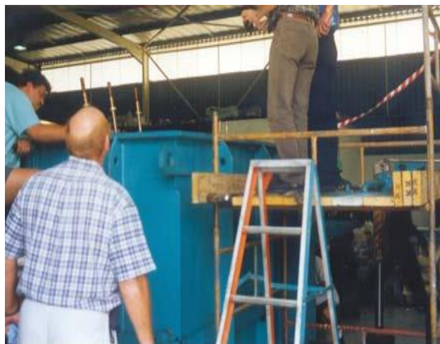
Figure 20: Reactor transformer being De-tanked at the Works facility
