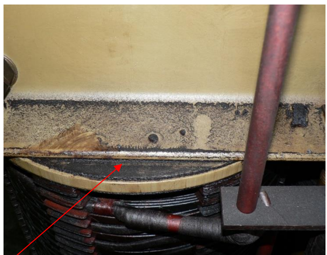
Residual Sludge By products of oil oxidation
