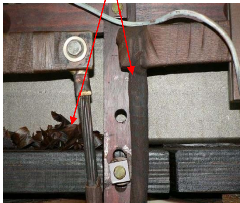
Extensive deterioration of the LV and Tap changer Leads
