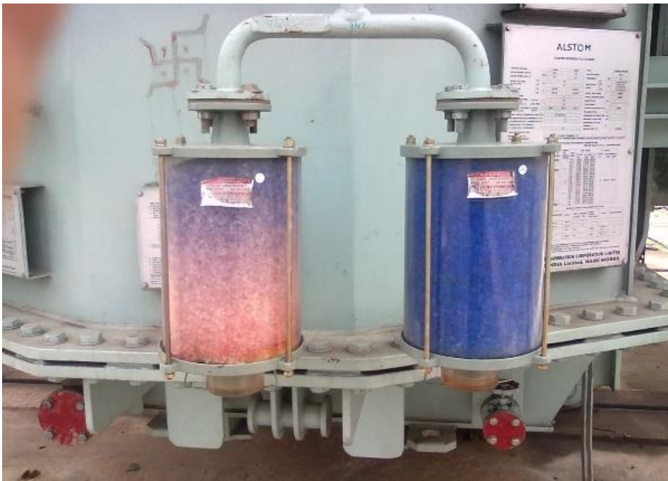
Figure 2 - Transformer breather
