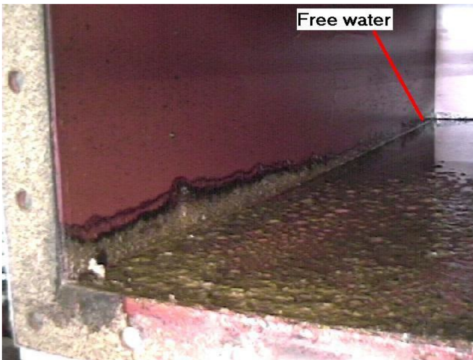
Figure 13 - Conservator tank
