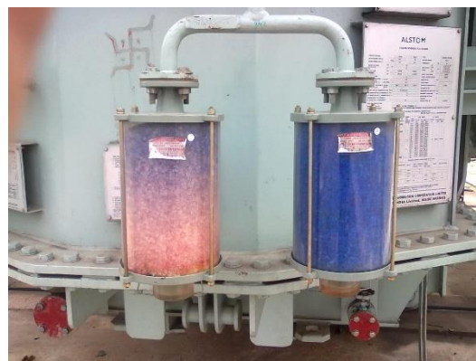
Figure 2–Transformer breather.
